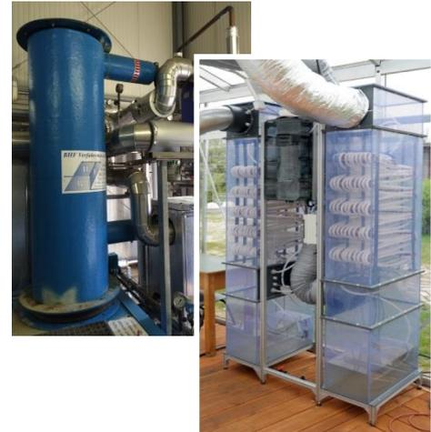
Figure 1: ZHAW and the project partner Watery tested the absorption technology in previous projects: the High Temperature Condensing Technology, installed by Bergmann (ZHAW) recovers heat from the flue gas in an ab- /desorption process (top); an absorption box of Watery is installed as air conditioner in a prototype building in (bottom)
